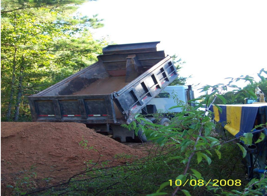
PHOTO 6: Placing of clean backfill in the excavated area
