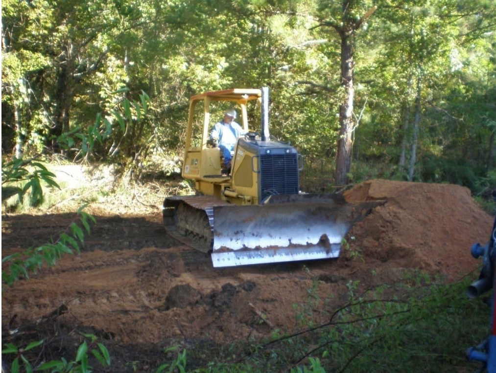
PHOTO 7: Spreading and compacting the clean fill in the excavated area
