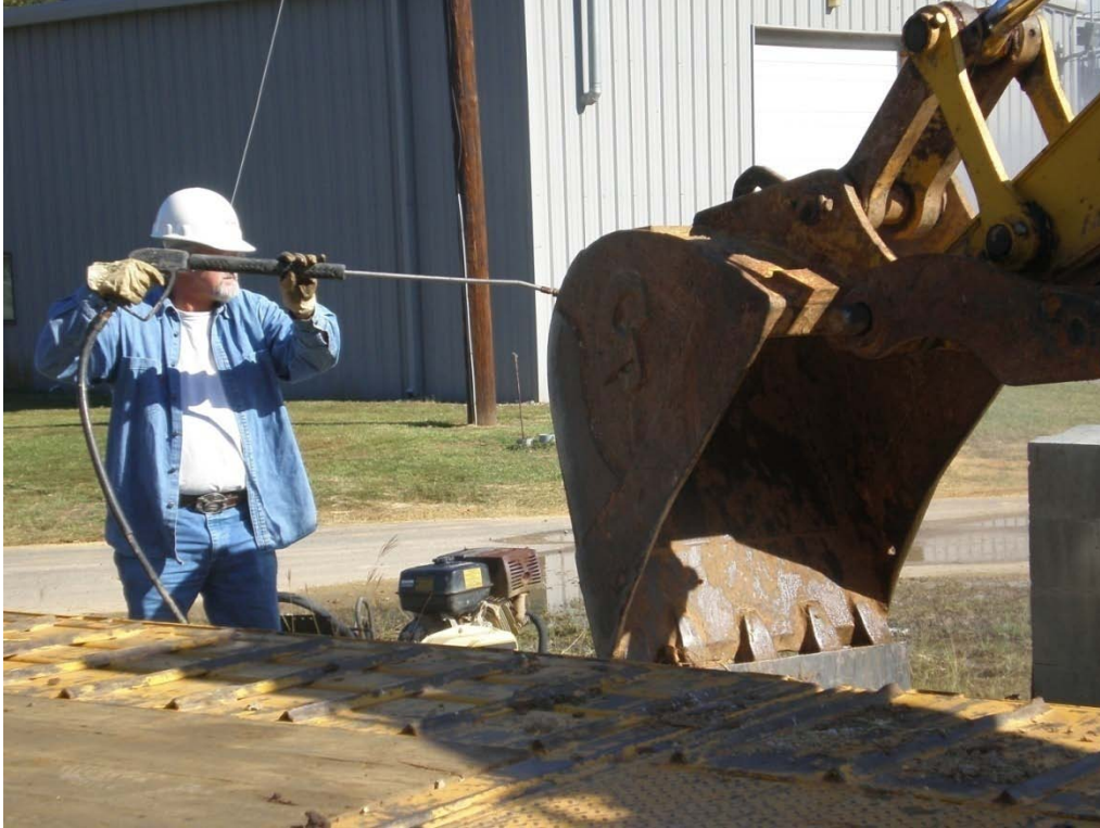
PHOTO 5: Decontamination of the trackhoe bucket using high pressure washer
