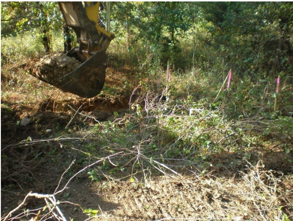
PHOTO 2: Removal of soil within the excavation limits
