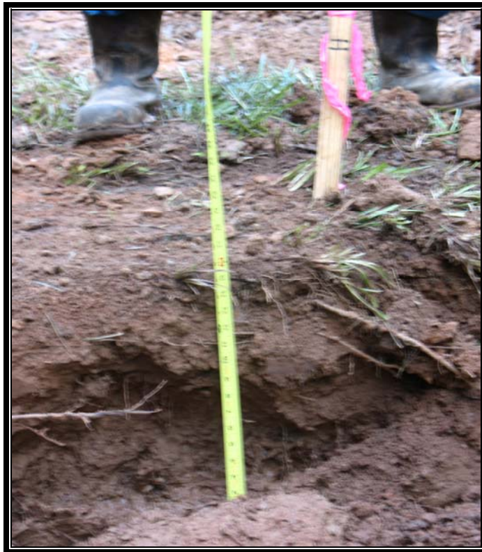
PHOTO 19: Exc. Depth Measurement – Stake H = 1.33 ft DATE: 8/7/09 VIEW: West
