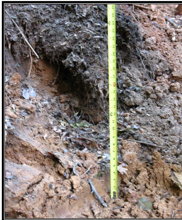
PHOTO 10: Exc. Depth Measurement – Stake C = 1.33 ft (Note: Stake not shown.) DATE: 8/7/09 VIEW: East
