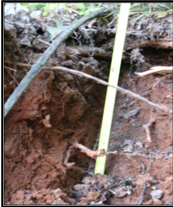
PHOTO 11: Exc. Depth Measurement – Stake D = 1.50 ft DATE: 8/7/09 VIEW: East
