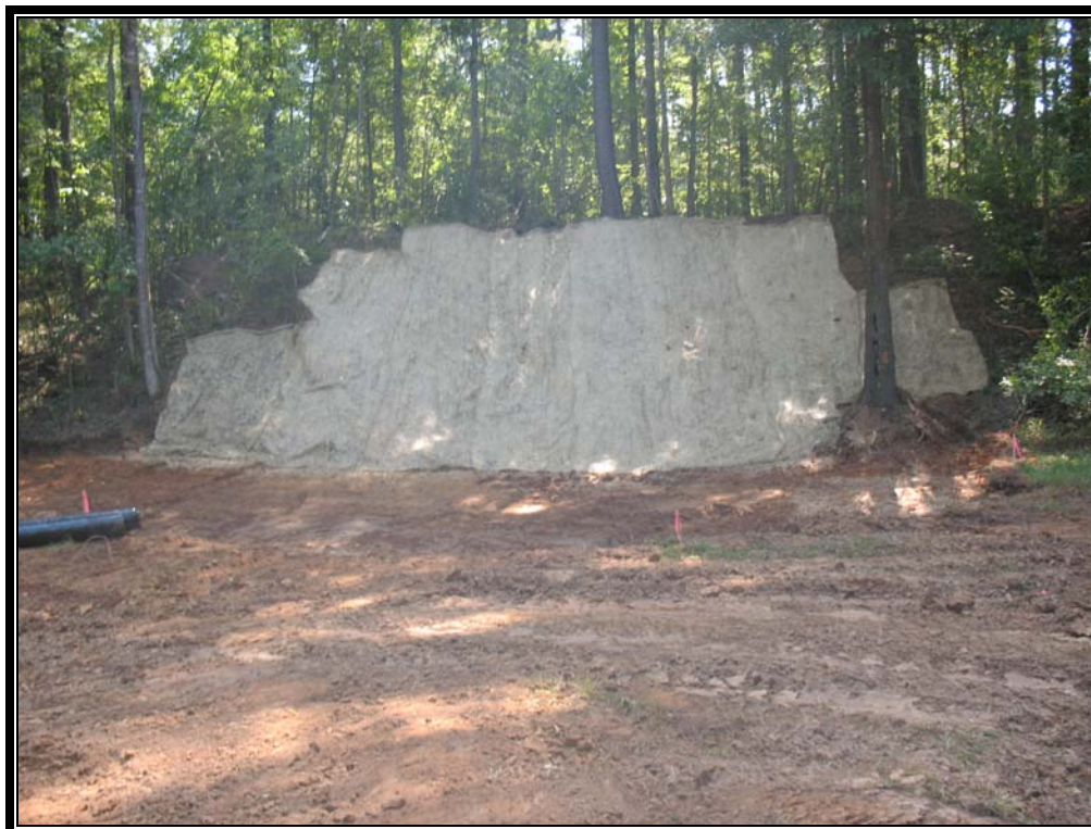
PHOTO 22: Erosion Control Straw Matting on Embankment DATE: 8/8/09
